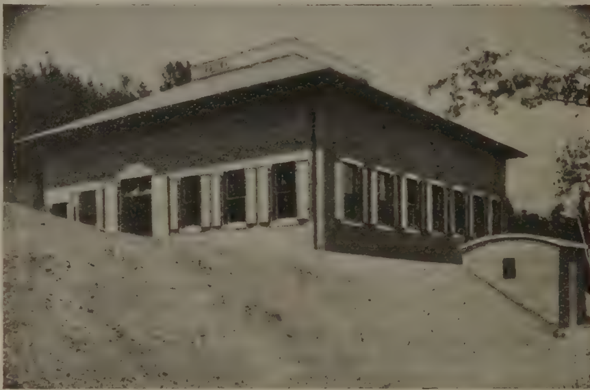
THE NEW PUMPING STATION AT GRAVEL POND
